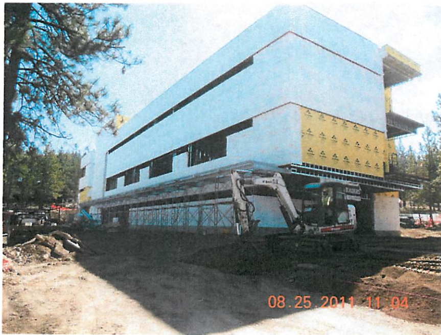
Building Wrap and Sitework
