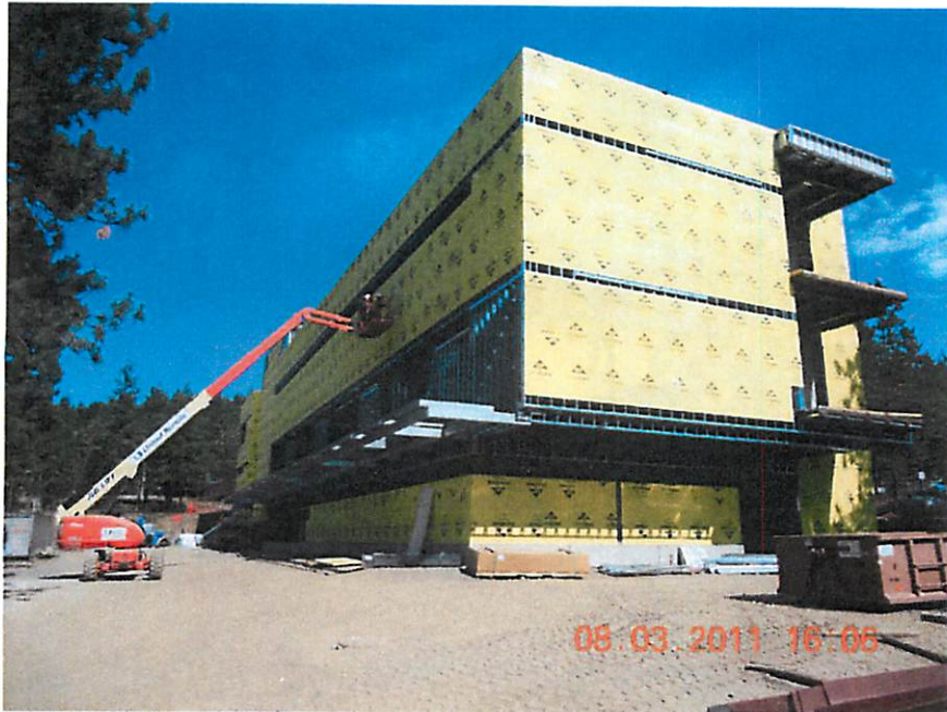
North Side Sheathing
