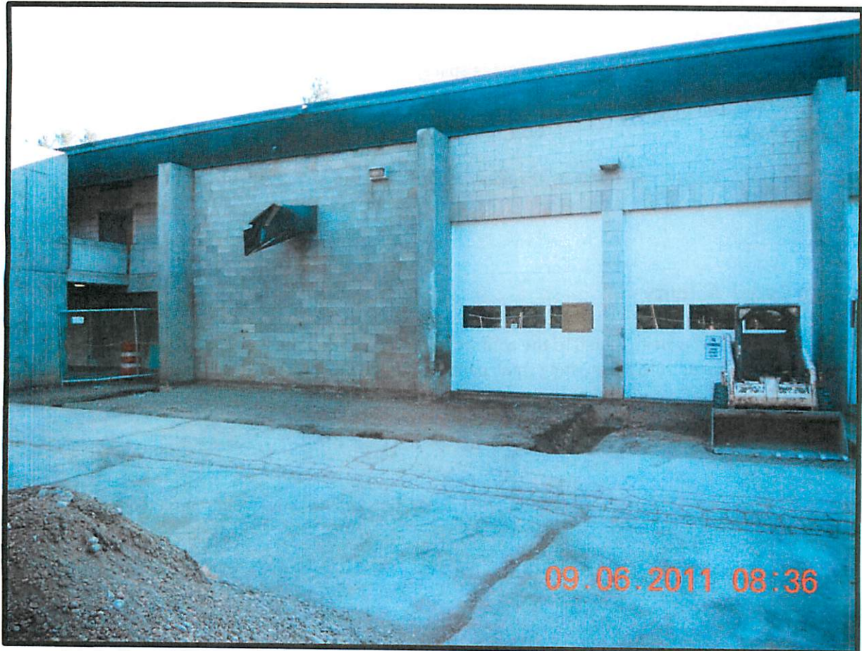
Masonry/concrete structure and fence removed. Foundation excavated.
