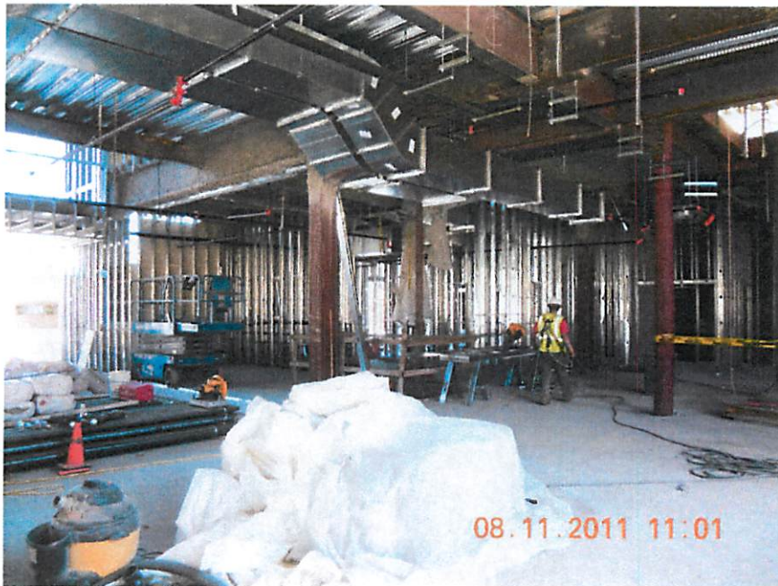
Interior Framing and MEP's Progressing
