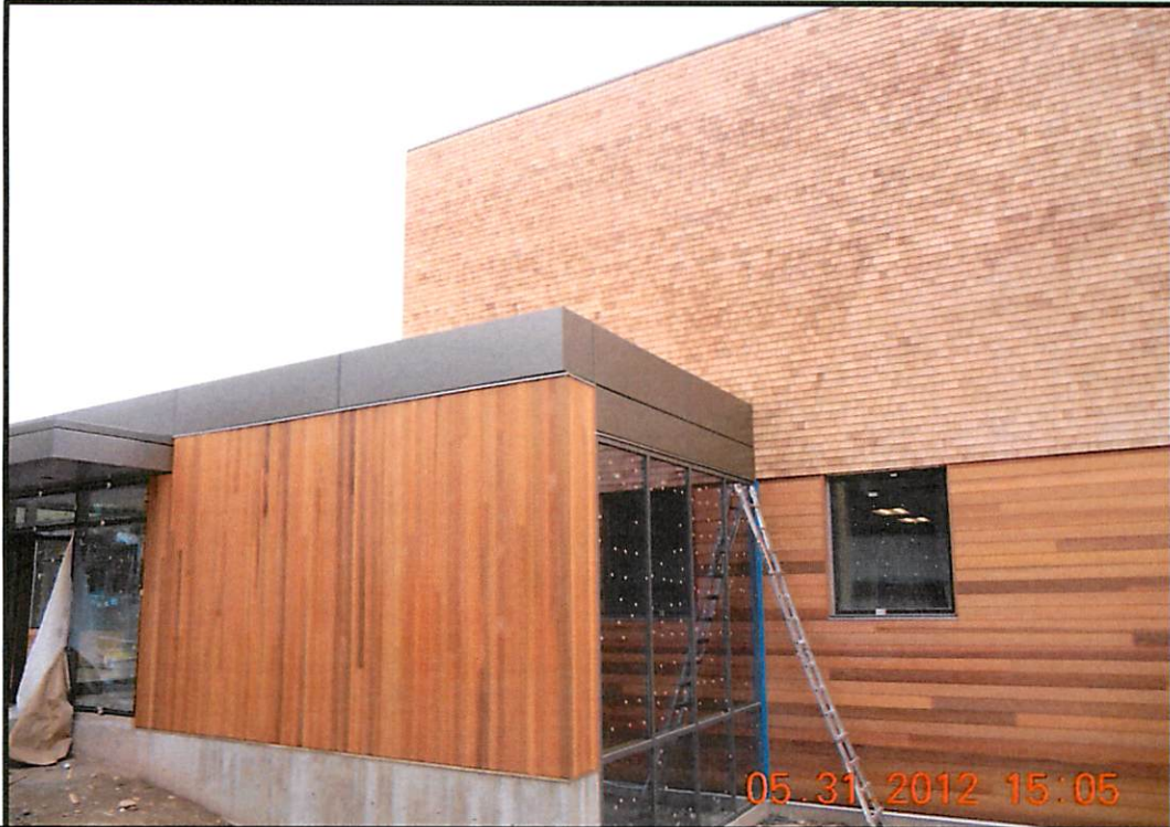
East Elevation: Glass and metal paneling substantially complete at SE vestibule.
