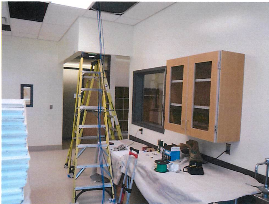
Camera and Speaker Wire Installation – Health Careers, Dental Assist
