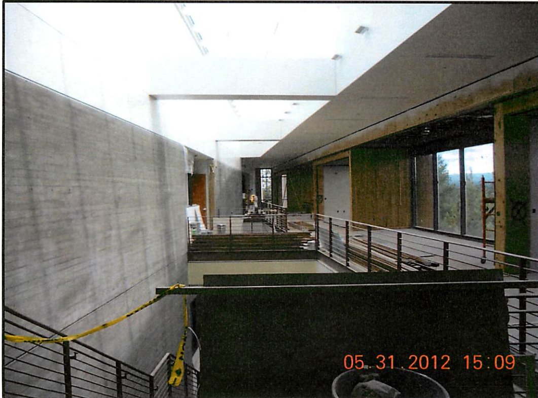
Second floor lobby/common area. Woodwork completed. Glass walls in progress.
