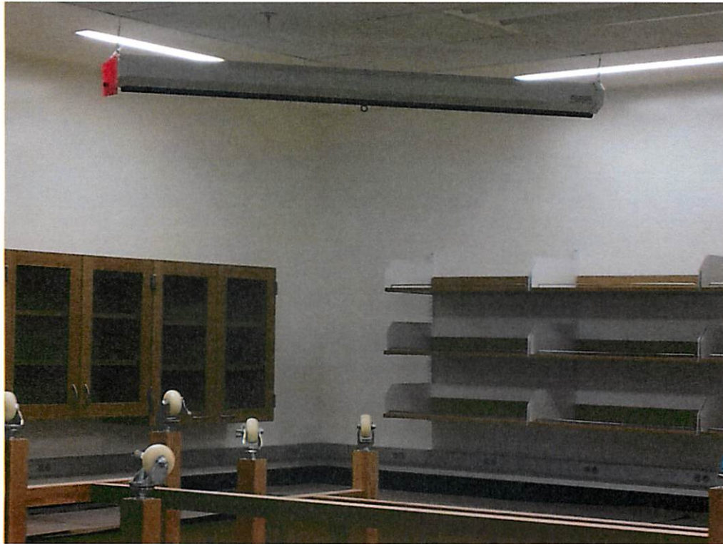
Projector Screen Installation – Science Building, Lab
