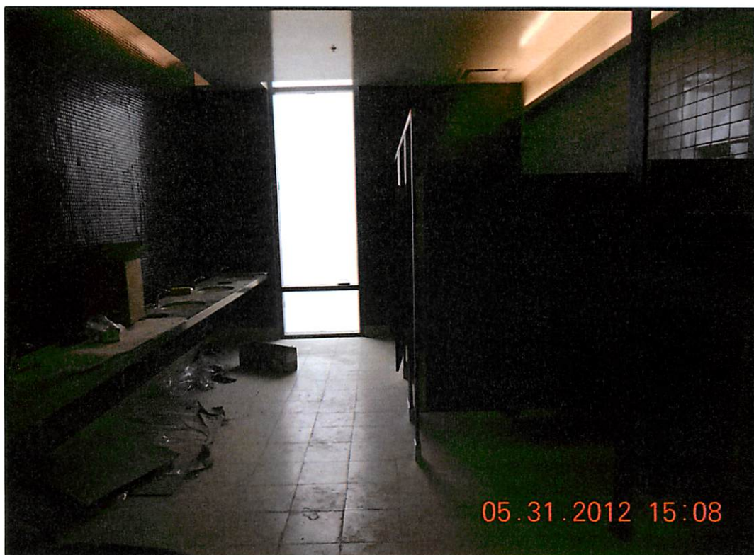
Second floor bathroom partitions and plumbing in progress.
