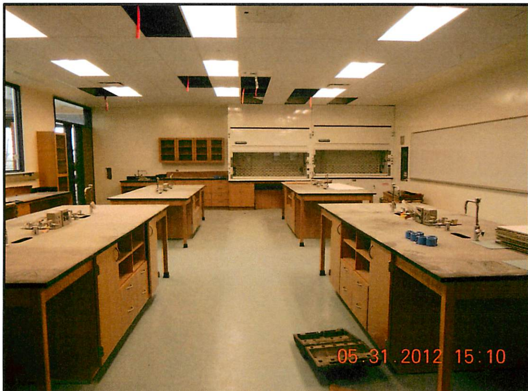
Chemistry labs in progress.
