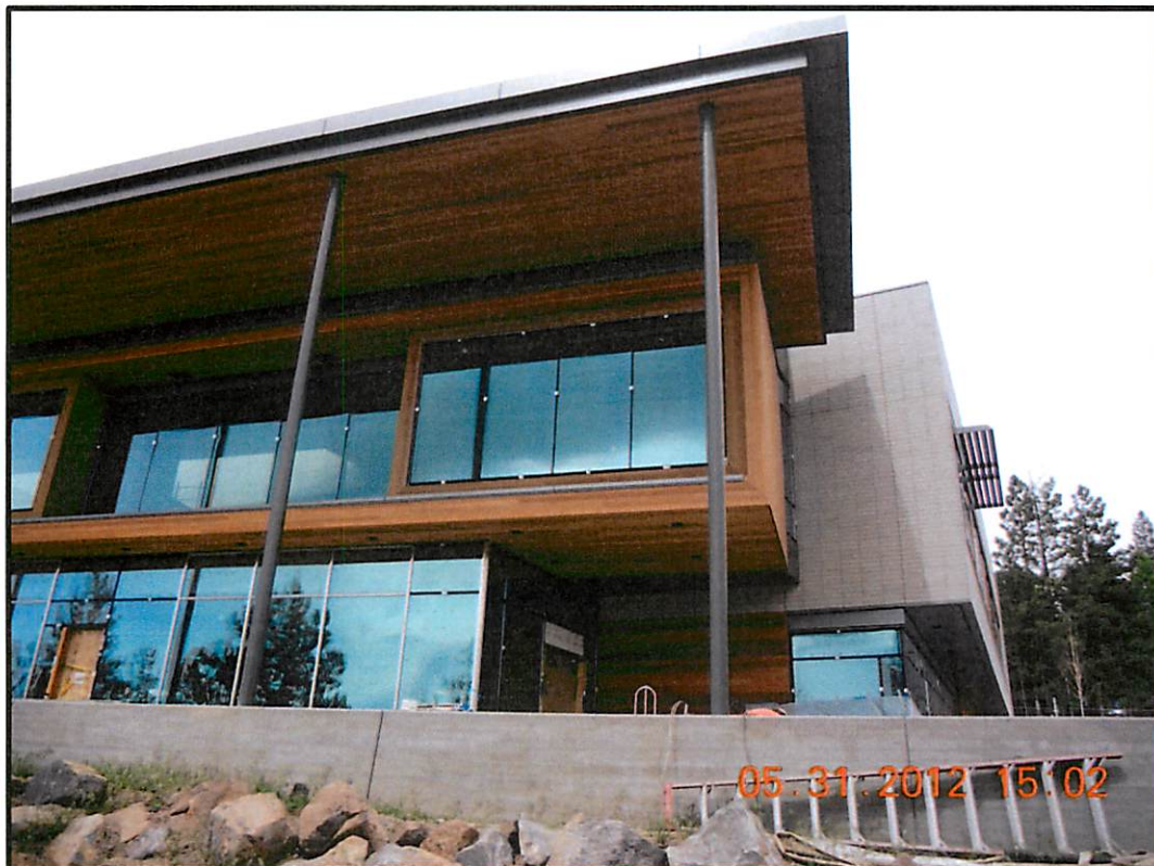
West Elevation substantially complete except doors, glazing caps, and light fixtures.
