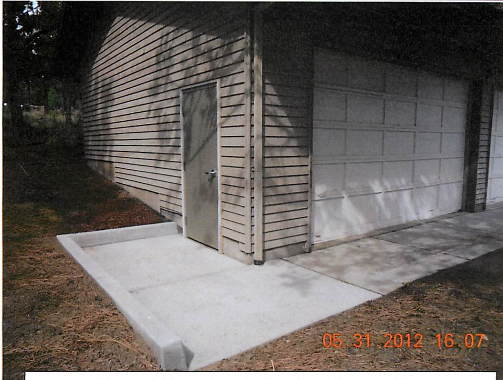
Garage division and exterior door installation complete.
