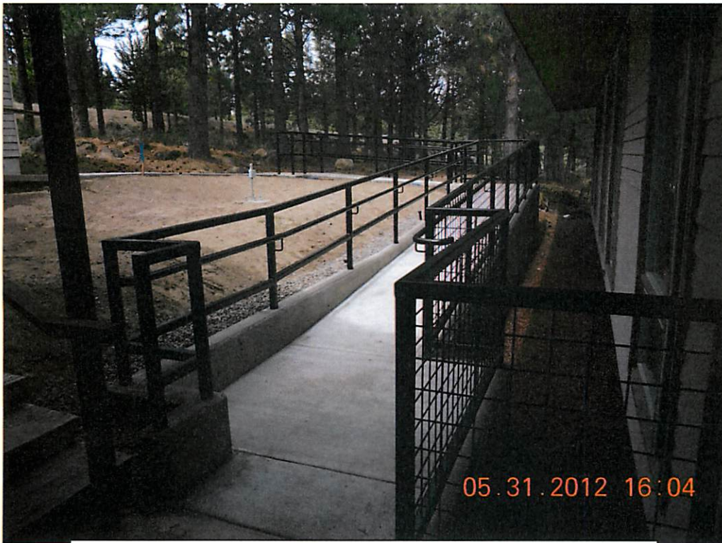
Ramp complete to upper meeting room.
