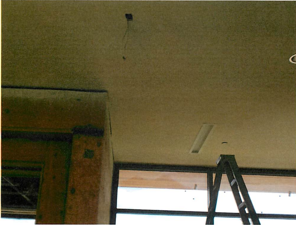
WiFi Access Point Installation – Science Building, 2 nd Floor
