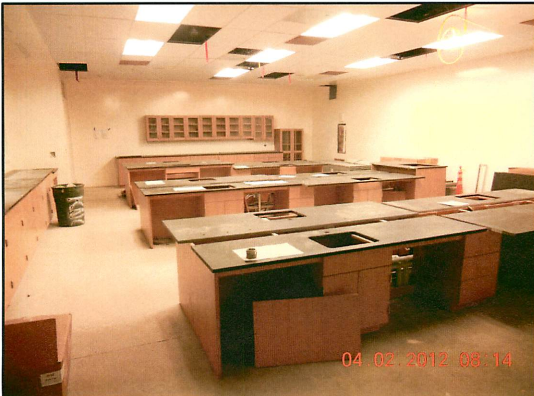
Biology Lab countertops installation in progress.
