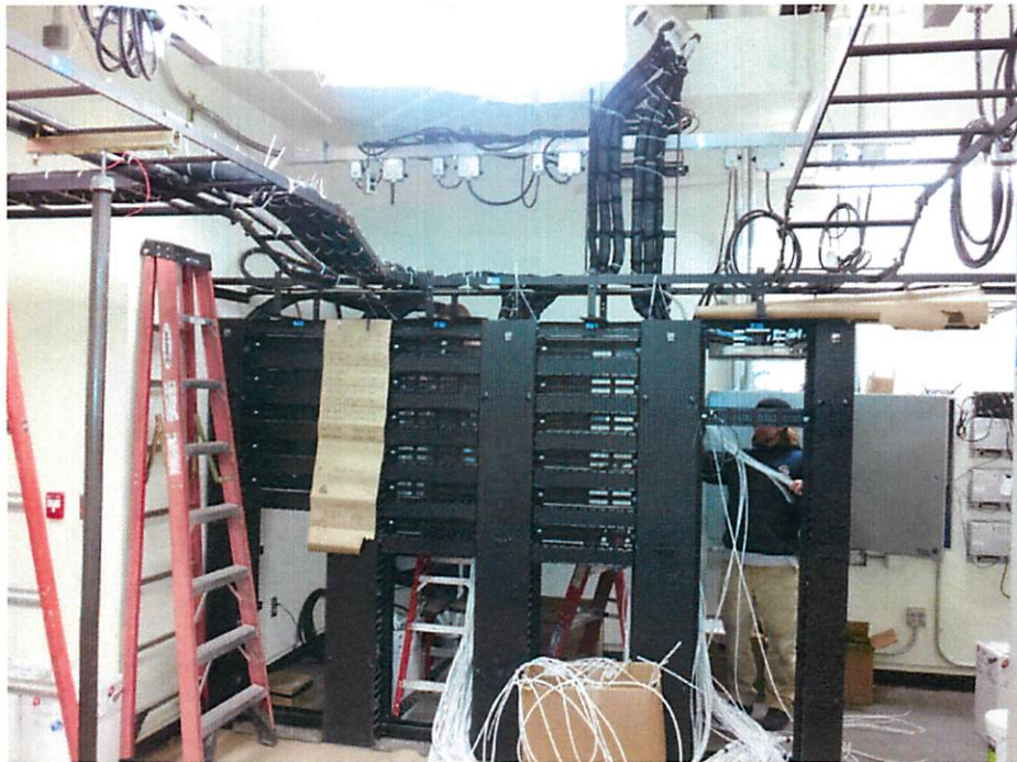
Racks & Patch Panel Installations – Health Careers, MDF
