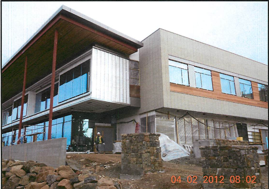
West Elevation glazing and metal paneling work in progress.
