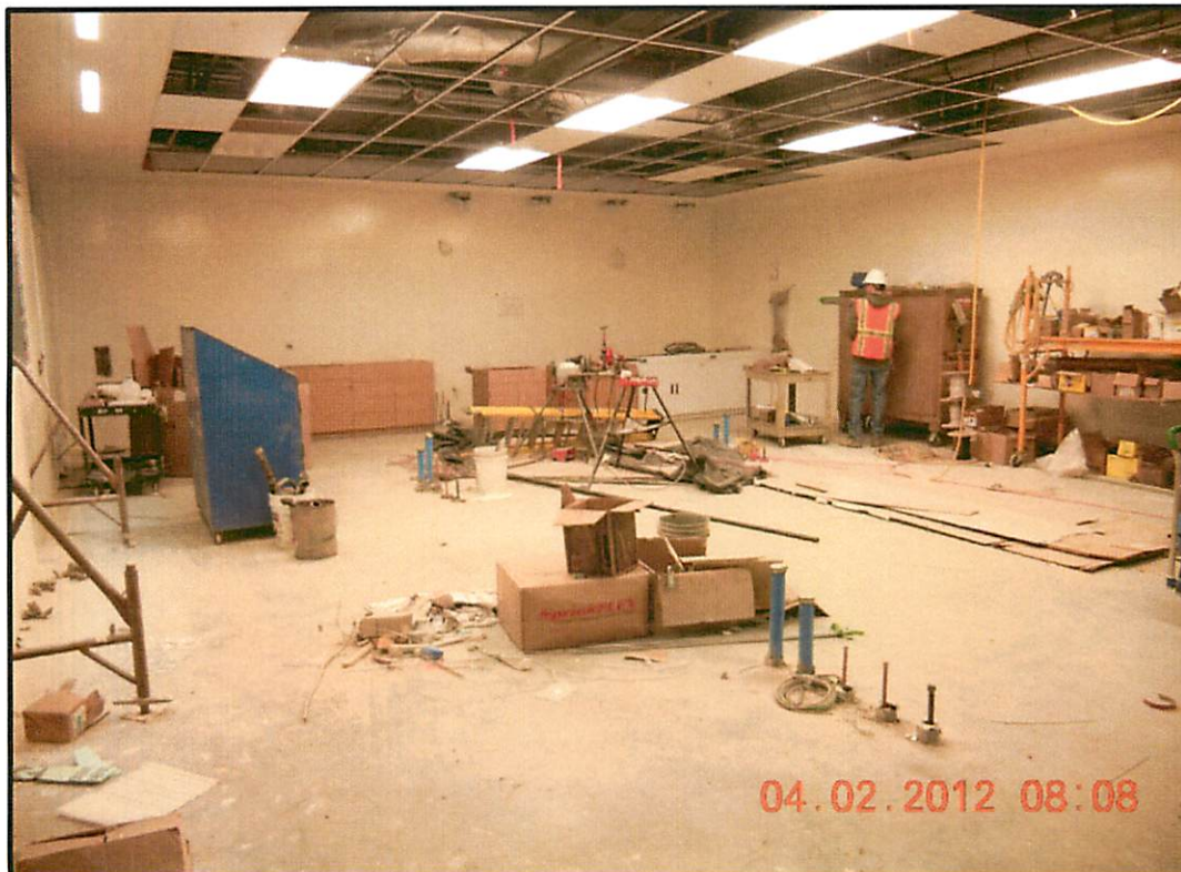
Chemistry lab casework installation beginning. Fume hood base cabinets in place.
