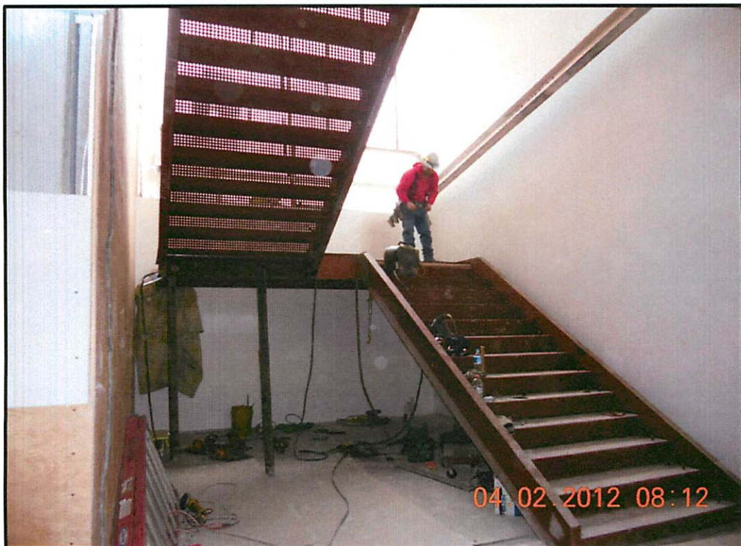
SE stairs installation progressing.
