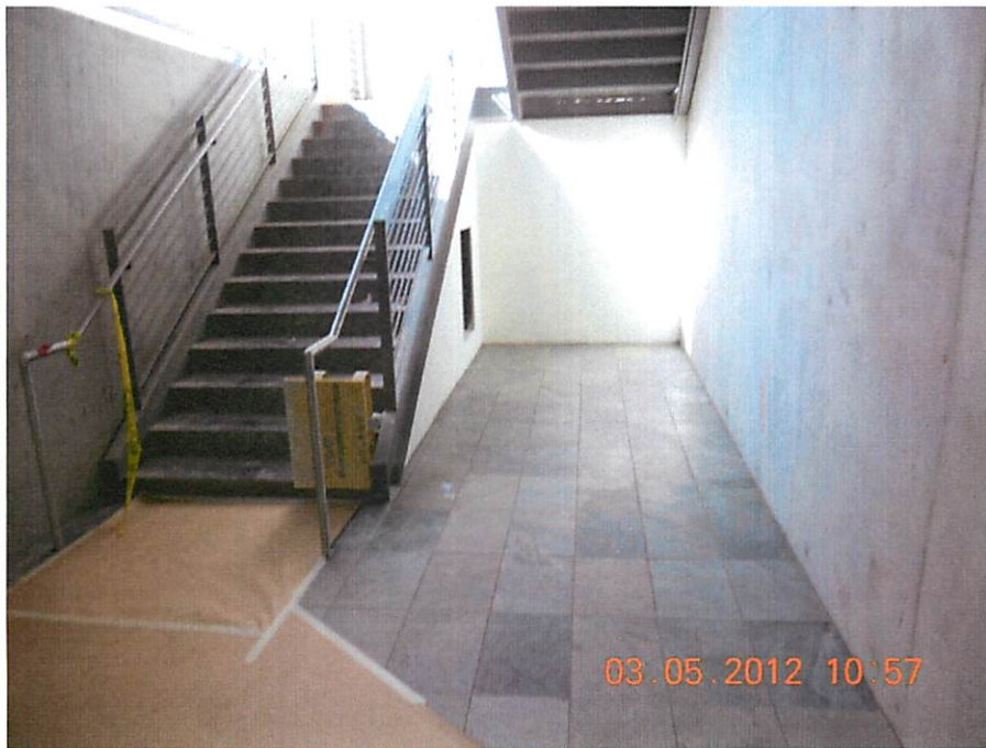
West Stairs – 1 st Floor
