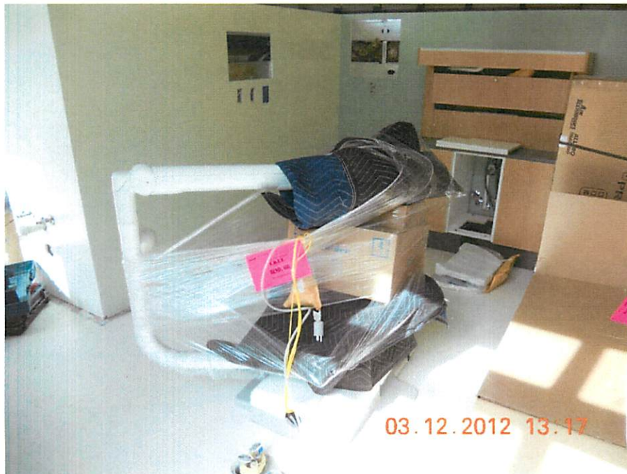
Dental chairs being installed.
