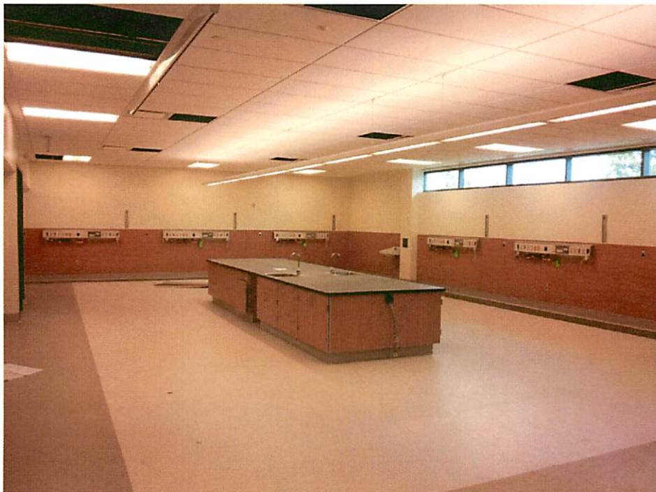
Installation of Nursing Headwalls – Health Careers, 3 rd Floor
