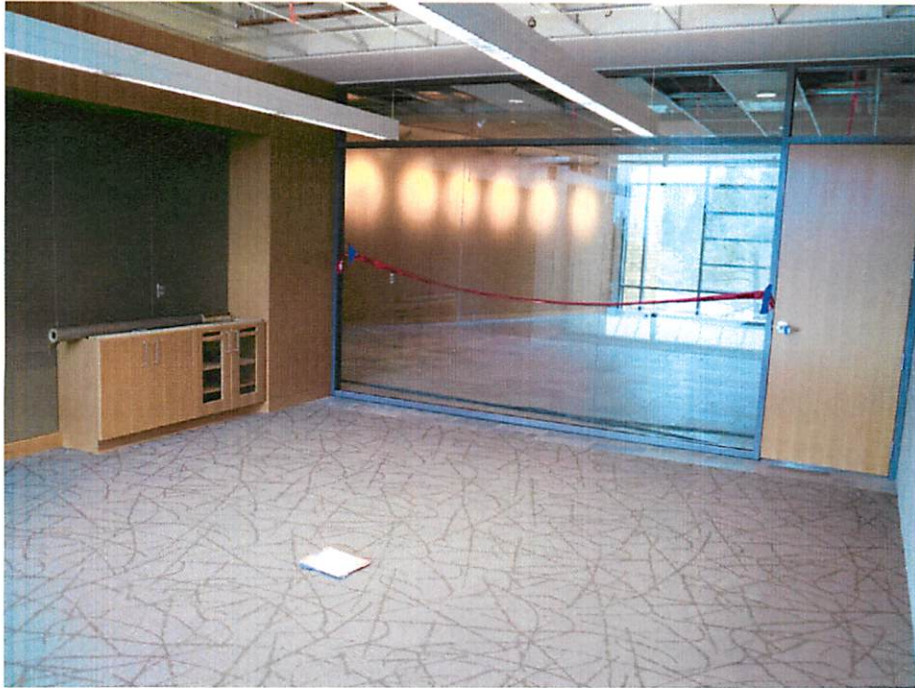
Installation of Audio-Visual Casework – Health Careers, Conference 301
