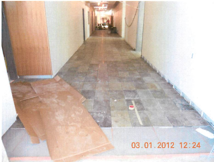
1 st Floor Hallway looking East from Main Door
