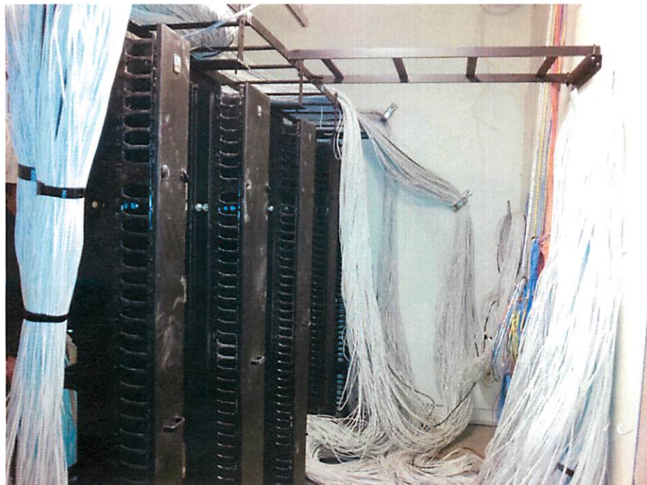
Cable & Ladder Rack Install – Science Building, MDF
