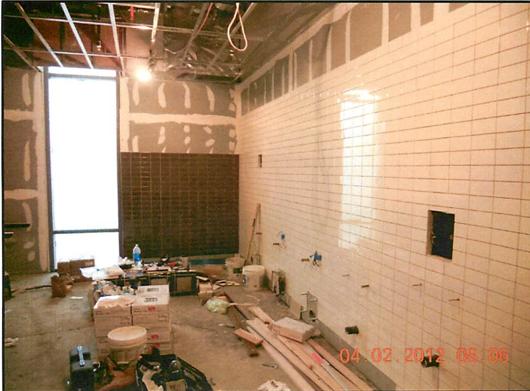
Second floor bathroom wall tile progressing.
