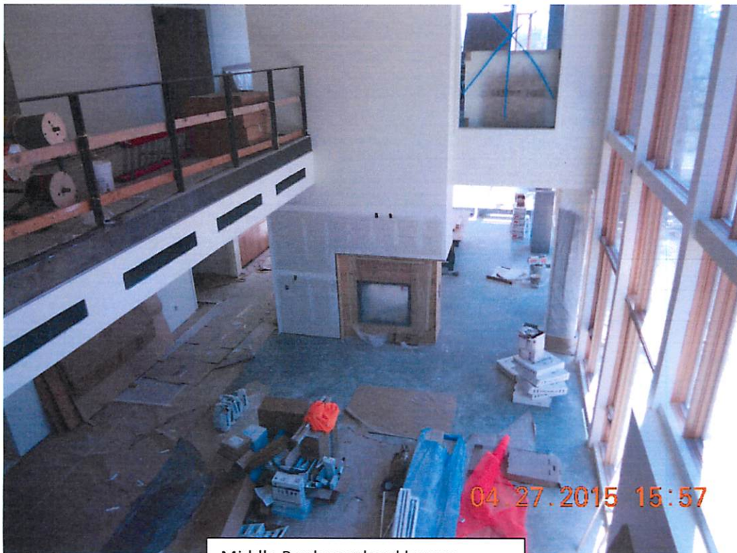
Middle Bar lower level lounge
