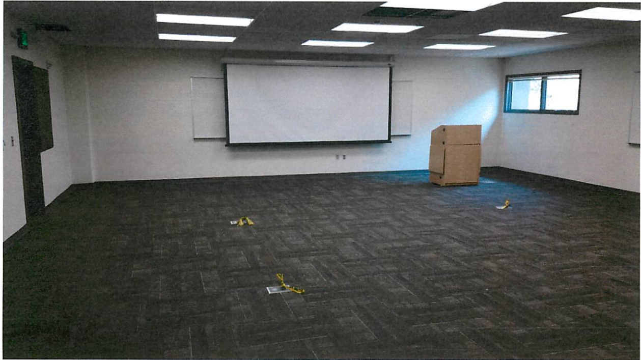
Projection Screen and Lectern Install – Ochoco, Computer Classroom
