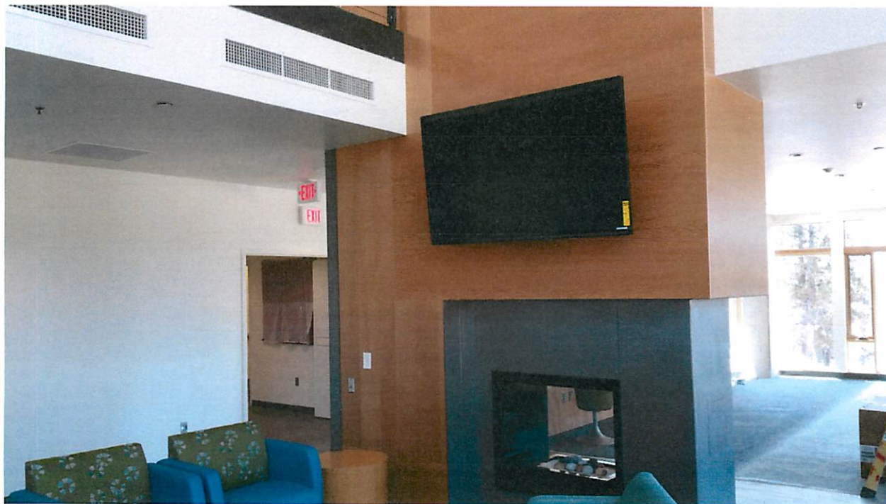
LCD Television Installation – Residence Hall, Lounge Area
