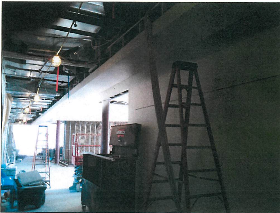
Data Cable Installation – Health Careers, 2 nd Floor Hallway
