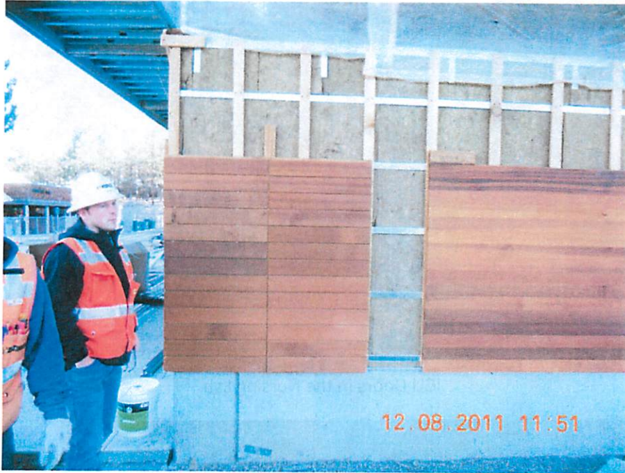
Painted vs. Bright head nail Mockup
