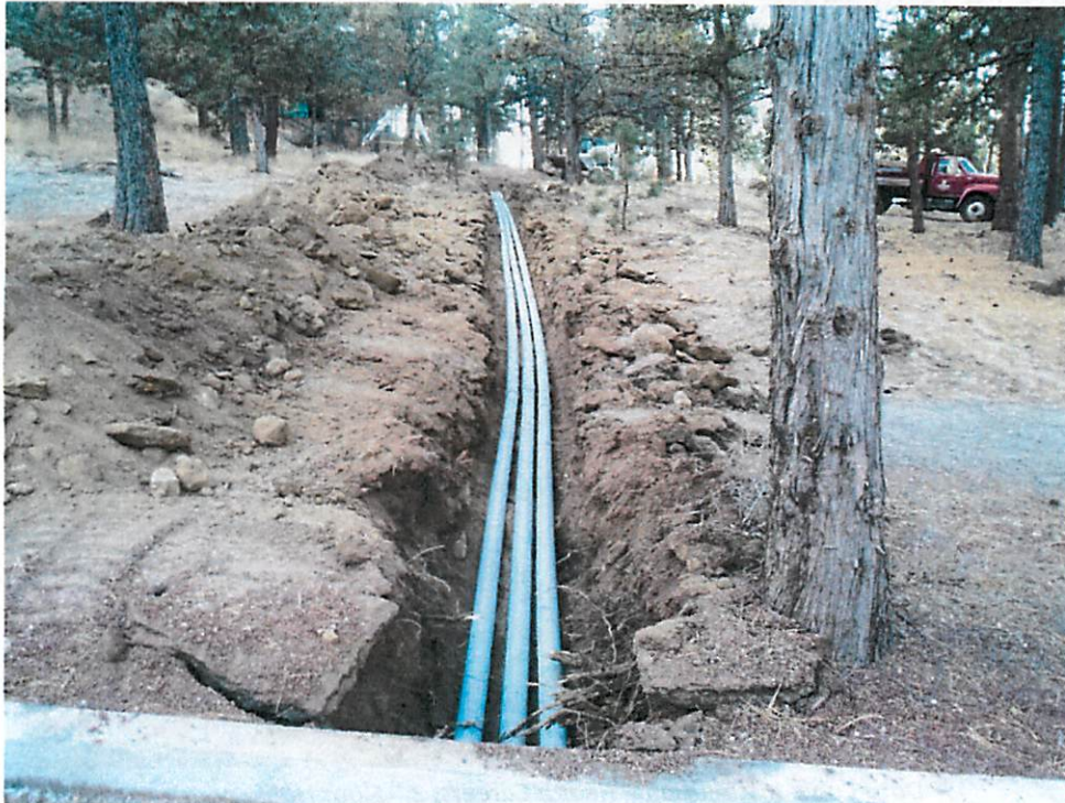
Fiber Conduit Installation – Health Careers, to Metolius
