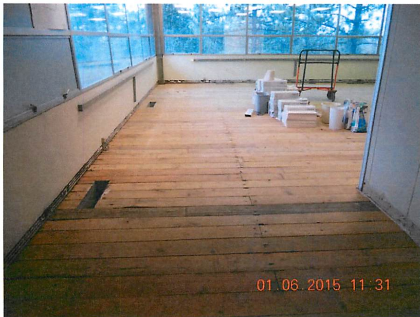
Room 232 after asbestos remediation.
