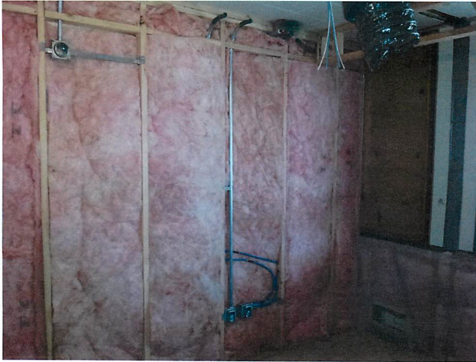
Power & Data Floorboxes – Typical Office, Ochoco remodel
