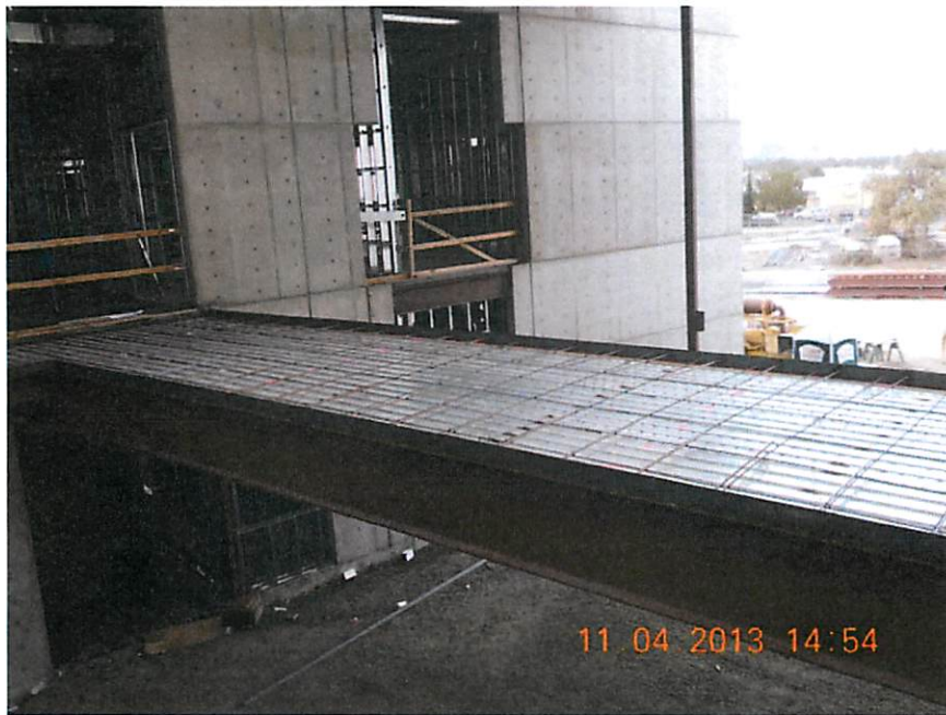
Looking into the Lobby from the 2 nd floor.
