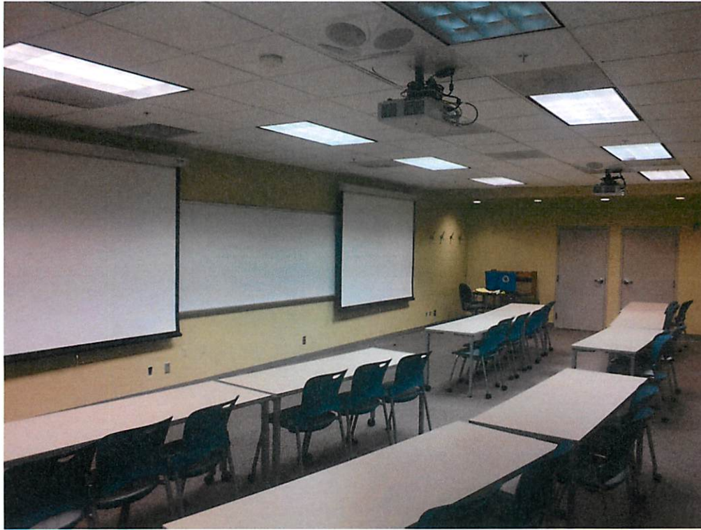
Dual Projectors & Projection Screen Install – Mazama 207
