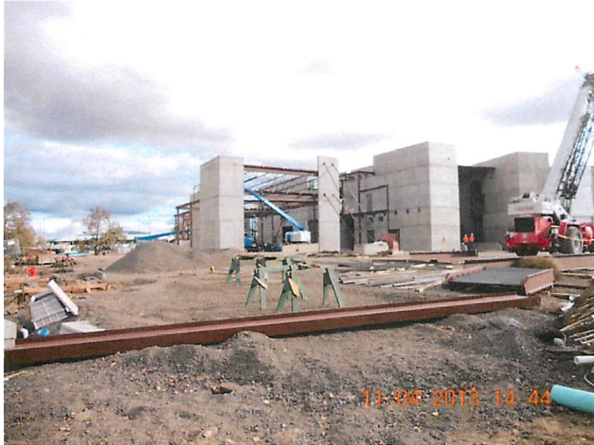
Setting roof joists.
