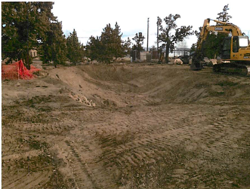
Along Airport Way – Storm-water Retention Basin
