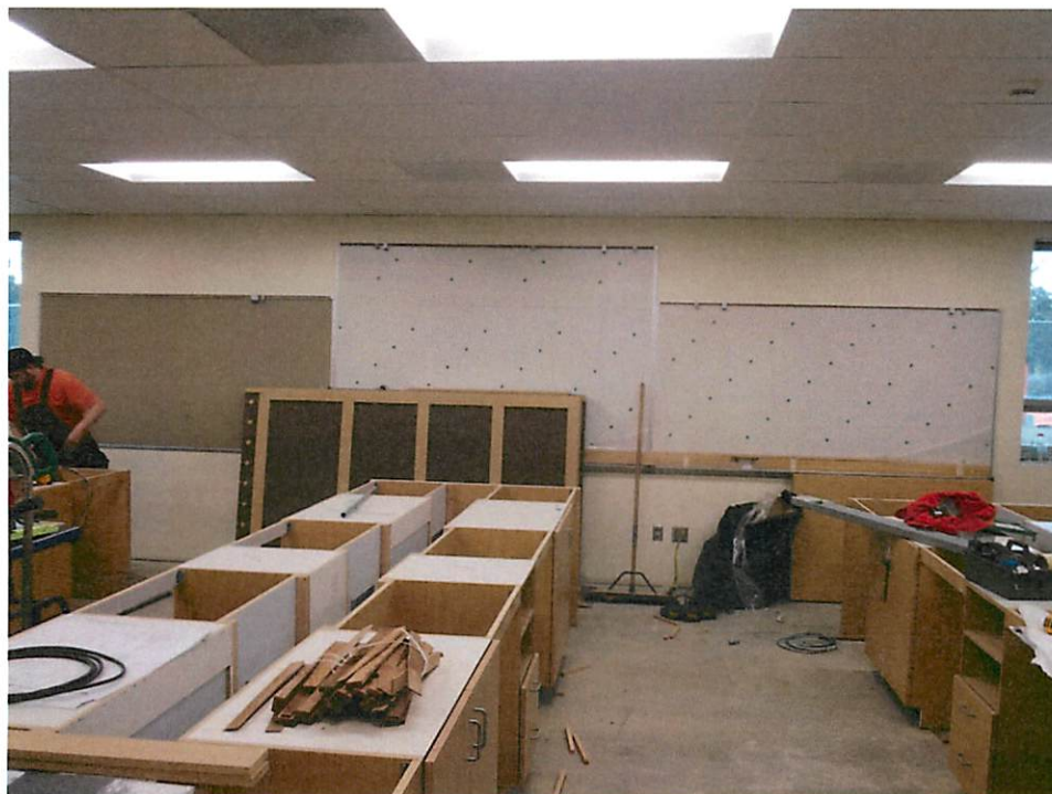
Whiteboards, Ceiling and Projector Tile Installed – Classroom 140, Redmond Building One
