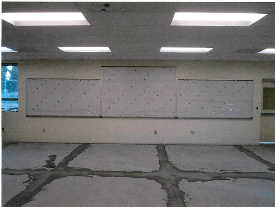
Whiteboards, Ceiling and Projector Tile Installed – Classroom 142, Redmond Building One
