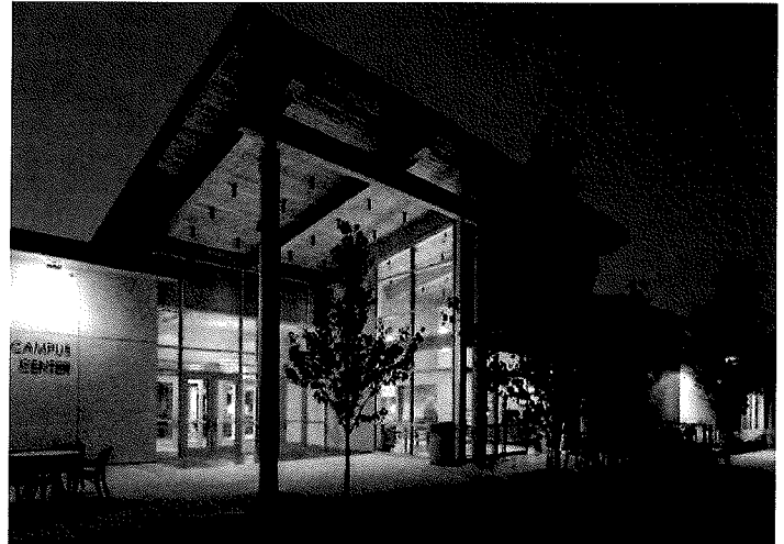
Design for high desert inclement weather encompasses consideration of durable systems and designs that address summer heat and sun, strong winds, fire season smoke, and winter snow loads.
