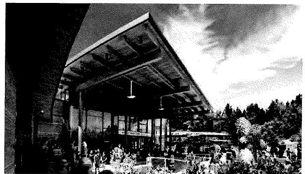
At the Net Zero Oregon Zoo Education Center, small things matter. This guiding principle is on full display from the expansive rooftop photovoltaic array, rain gardens that clean stormwater before reuse in restrooms, and bird-friendly lighting and fritted glass windows.
