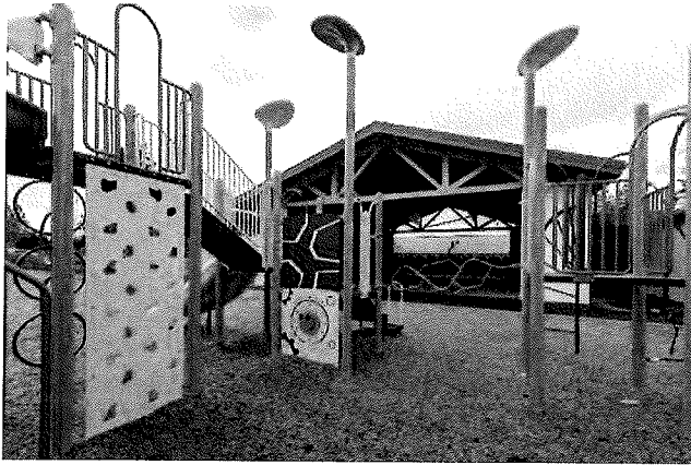
El Puente Elementary School - Two conditioned corridors now connect the previously detached kindergarten classrooms and a taller, more functional covered play area was built in between the corridors.
